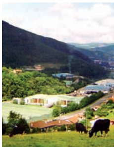
Gerflor Tarare manufacturing plant
