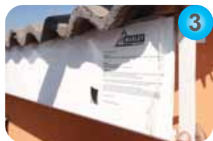
Attach Fascia stopend Peel back protective layer back slightly to attach stopend
