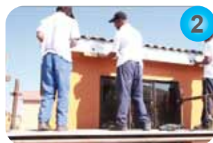
Fit Fascia Ensure the fascia is level. Fix with non-corrosive fixings
