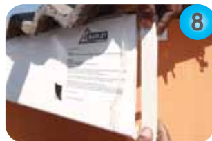
Fit Stopend Peel back protective layer slightly & fit stopend
