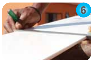
Measure next length Mark with a square
