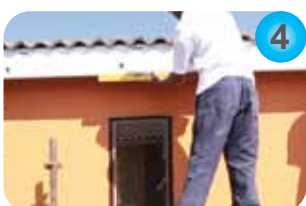
Check Fascia is straight Use a spirit level
