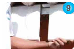
Join the two Fascia boards Peel back protective layer from second fascia & connect
