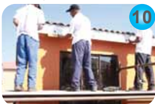
Fit Fascia Fix with non-corrosive screws every 750mm
