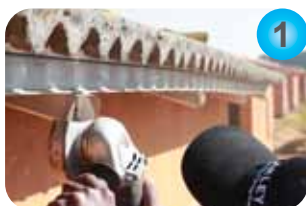
Trim rafters/ends Ensure straight finish
