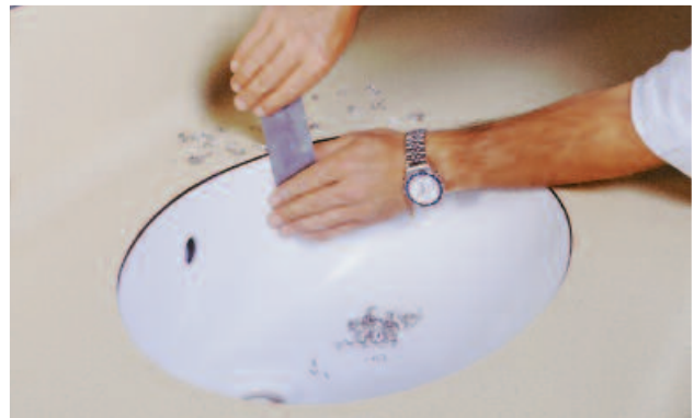
5. Fine clean and finish off with a scraper and sandpaper.
