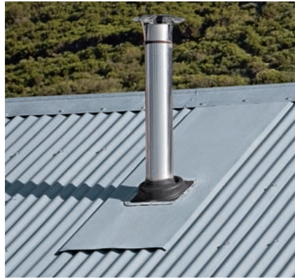
View of chimney penetration with flashing
