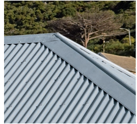
View of Ridge and Hip Flashing
