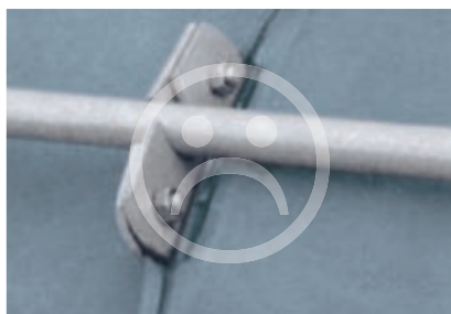
Snow guard system The clamp has to allow thermal length expansion of the pipe.
