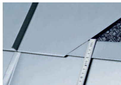
Cross joint designed as a single seam
