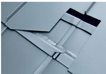
Detail optimization: soldered continuous cleats
