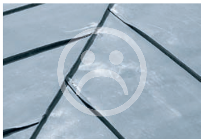
Hip or ridge designed as a double standing seam
