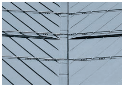
Valley gutter recessed on structured mat
