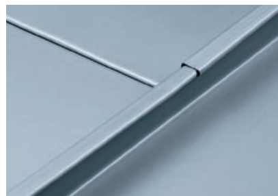
Seam in seam cross joint for angled standing seam system
