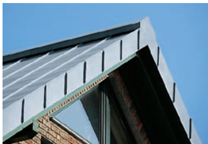
Ridge for a vented gable roof – high design with ventilation cross-sections
