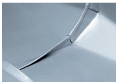
Double pinched seam in cross joint (3) Back apron
