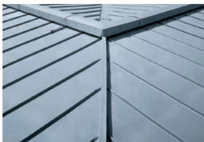
Hip with batten and coping profile
