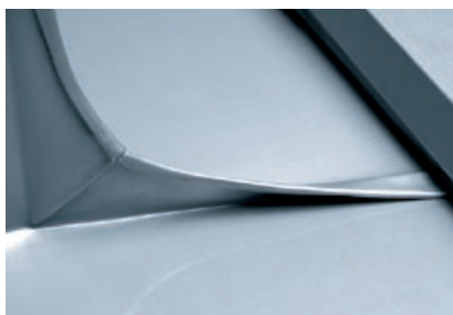
Rounded seam connection (1b) As 1a, but seamed to expansion strip
