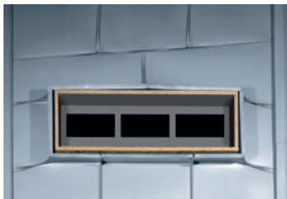
Roof penetration Details: proper seaming technique design (drawing – see page 12)
