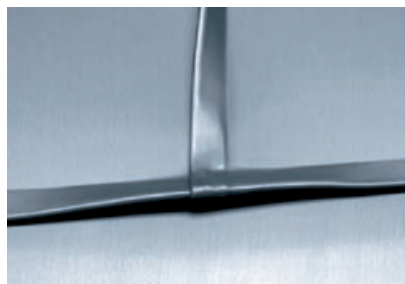
Intersection (4) Panel on cross joint, back apron
