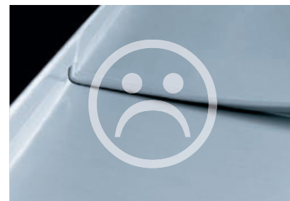
Gable roof ridge without expansion area and insufficient installation height
