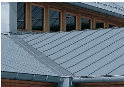
Valley with a single seam and soldered continuous cleat
