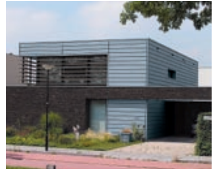
Private Residence, Empel, Netherlands
