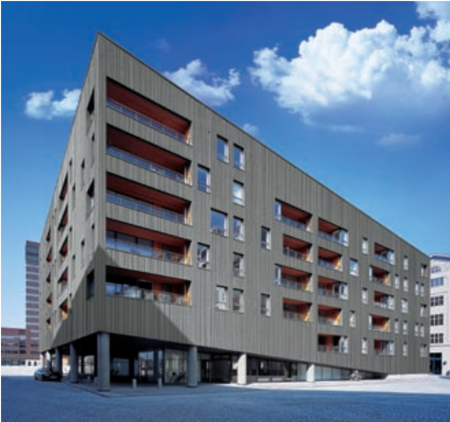
Zinkhaus, Copenhagen, Denmark
