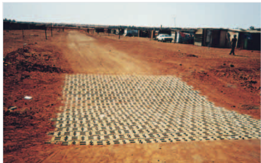
Armorflex lined stormwater crossing of gravel and surfaced roads
