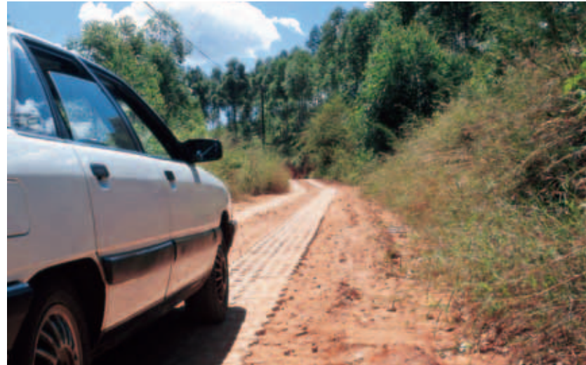
Armorflex as strip road in forest area
