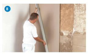
Tap the board back firmly using a straight edge until it butts against the top and bottom angles.
