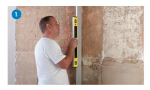
Determine high spots on the wall and plumb position to the ceiling and floor.
