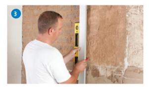
Mark wall with lines at every 1200mm centres to indicate board positioning.
