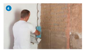
Trowel apply a continuous fillet of Gyproc RhinoLite or Gyproc RhinoBed (new) to the perimeter of the wall surface and openings where required.
