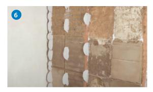
Position dabs of RhinoLite on three vertical rows (at 600mm centres) to receive the first board. Ensure that the dabs adjacent to the board joint are approximately 25mm in from the edge to avoid bridging the joint.
