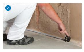
Transfer this dimension to the room corners. Add an allowance of 10mm plus the thickness of the Gyproc RhinoBoard and strike continuous chalk lines on the floor and ceilings. Fix Donn Galvanised Steel Angle 20x20mm.
