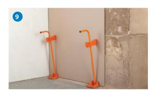
Gently lift using foot lifters until the board is tight against the ceiling. Apply dabs for the next wallboard and continue the dry lining with boards lightly butted.
