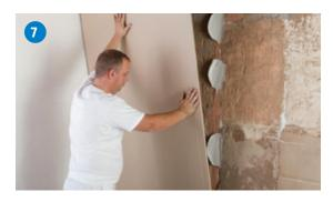
Cut the RhinoBoard 15mm short of the floor to ceiling height. Position the first board printed side against the dabs, with the bottom edge resting on the plasterboard packing strips/board lifters.
