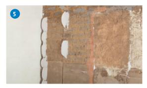
Commence dry lining from a window/door reveal or internal angle. Trowel apply RhinoLite or RhinoBed to form dabs 50mm to 75mm wide and about 250mm long.
