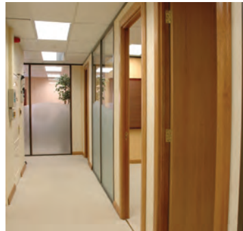
Main Post showing partition board and centre glazing details.
