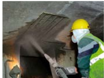
Repair, protection and strengthening of concrete
