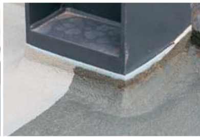
Floor connection joints
