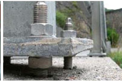
Anchoring; bonding of threaded rods and rebars
