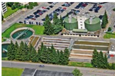
Sewage water treatment plants
