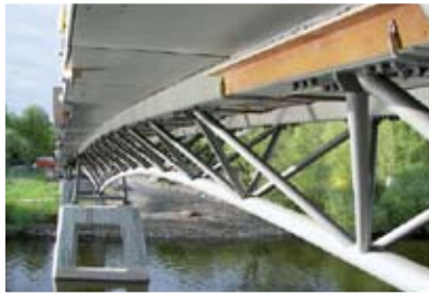
Bonding of bridge elements
