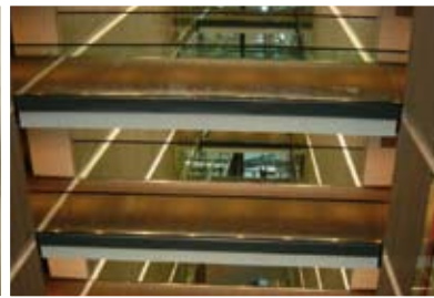
Glass panel grouting
