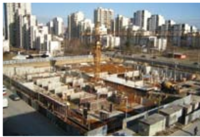
On site concrete production
