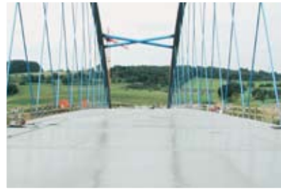
Bridge deck waterproofing
