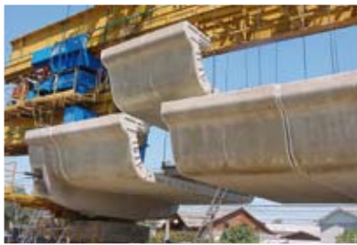
Precast concrete industry
