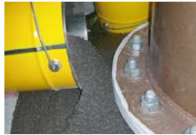
Epoxy resin grouting
