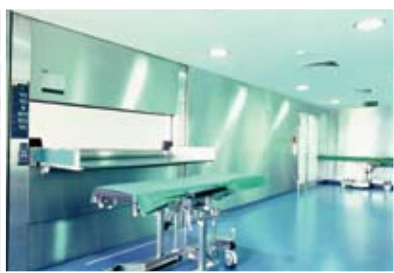
Clean room environments
