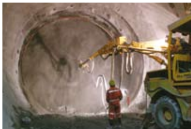
Sprayed concrete applications
