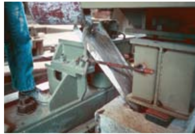
Machine base plate grouting
