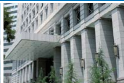
Weather sealing of natural stone façades
