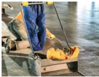
Flooring, coating and wood floor bonding
