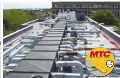
Roof refurbishment with liquid membrane
