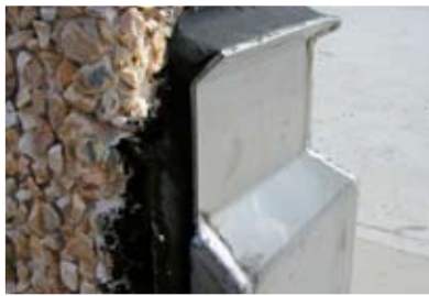
Roof connection joints
