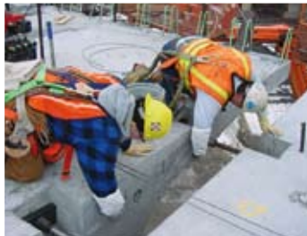
Structural bonding and grouting
