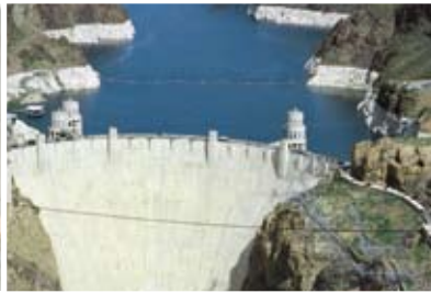
Structural bonding in dams
