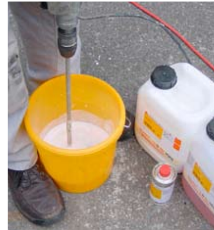
Mixing of an acrylic injection resin
