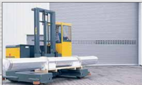
The shutter curtain can be placed onto pre-assembled consoles by a forklift truck.
