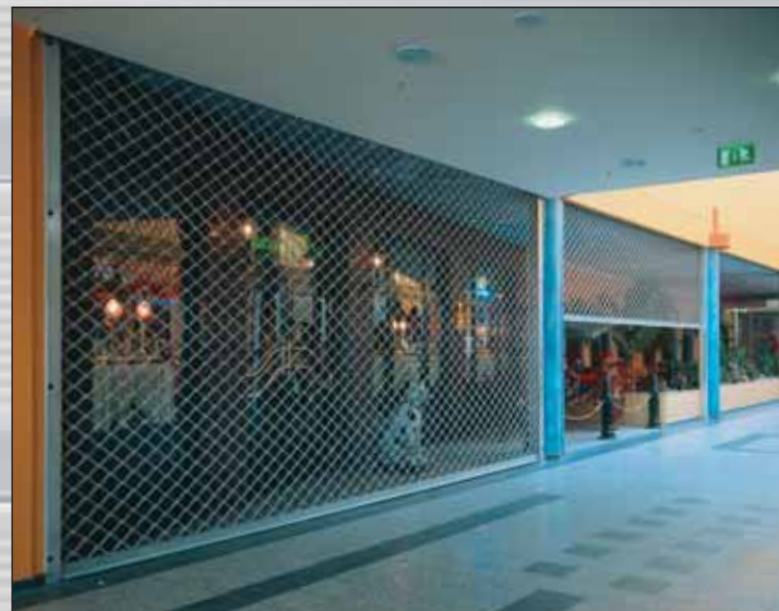
Shop front security.
