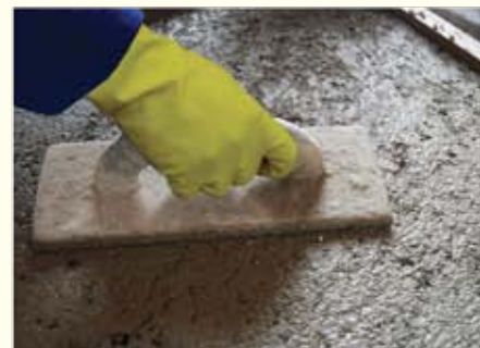
Wood float the surface. DO NOT add extra water during this process
