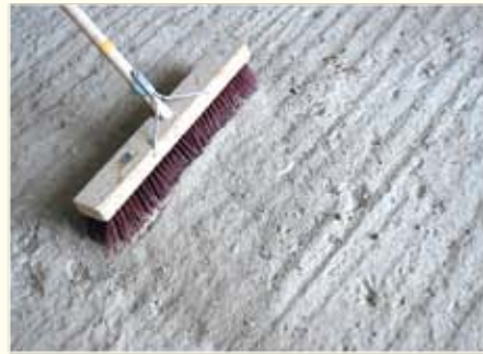
Sweep the floor to remove all dust and debris
