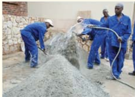
Add water to obtain a stiff consistency
