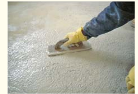
Wood float the Grano Colour into the surface
