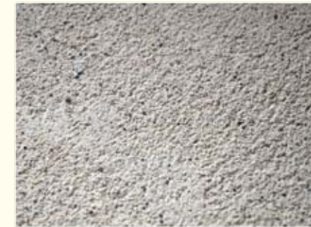
Leave to soak up the water from the screed
