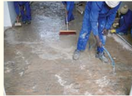
Flush clean with water and remove all loose material using a hard bristle broom
