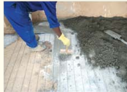
Mix equal volumes of plaster sand and OPC. Add Weber Key-it to create a creamy, brushable slurry. Apply to the base concrete using a block-brush
