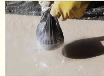
To obtain a smoother surface, sift Grano Colour through a very fine sieve or stocking to remove all coarse material and apply to the wet surface
