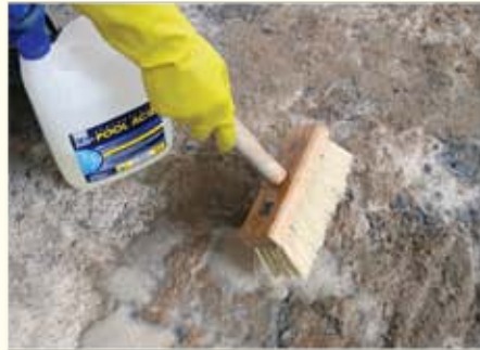
Combine 3 volumes of water and 1 volume of hydrochloric acid in a plastic bucket and apply this solution liberally to the base concrete
