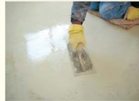
Steel float immediately to obtain a smooth finish
