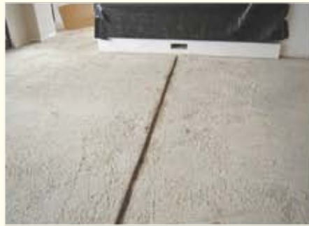
Expansion joints must be cut before application commences
