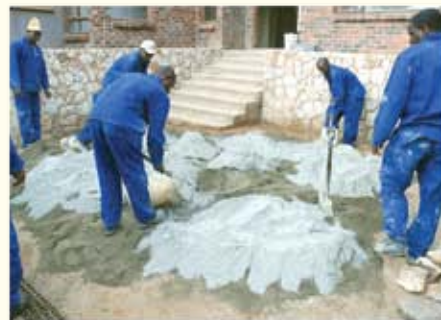
Combine 4 volumes of crusher dust or clean river sand with 1 volume of 42.5 cement
