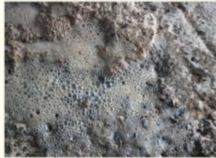
Wire-brush the surface vigorously and then allow the acid solution to react for a further 15 minutes
