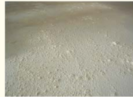
Apply Grano Colour by dry-shake method at a rate of 5kg/m 2 directly to the surface of the entire screed
