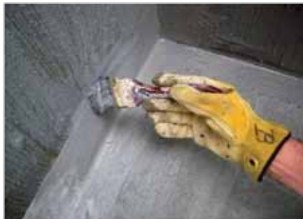
Apply Part C onto the wet slurry and press down firmly. Allow the membrane joints to overlap by 100mm with neighbouring membrane. Brush out any air pockets. Immediately apply a second coat of slurry, ensuring that Part C is completely saturated.
