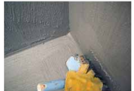
Apply a 1.5 to 2mm thick coat of the Part A/B slurry to all corners of the shower cubicle using a block-brush. Allow returns of at least 100mm to accommodate the bedding of part C.
