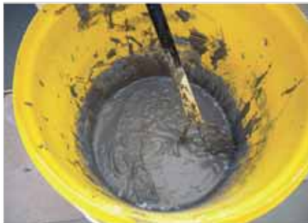
Combine the two bags of Part A with Part B and mix to a creamy slurry. Allow the mixture to mature for 5 minutes. Do not add more water.
