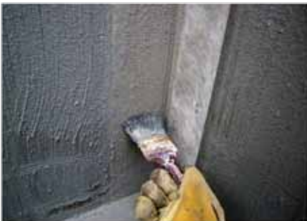
Apply Part C onto the wet slurry and press down firmly. Allow the membrane joints to overlap by 100mm with neighbouring membrane. Brush out any air pockets. Immediately apply a second coat of slurry, ensuring that Part C is completely saturated.
