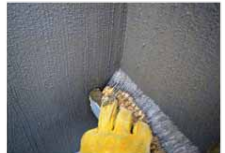
Apply a 1.5 to 2mm thick coat of the Part A/B slurry to the rest of the walls and floor of the shower cubicle. Ensure that they are well coated with no visible background showing through. Allow to dry for 24 hours before tiling commences.
